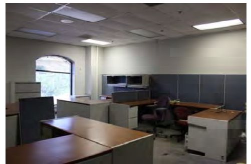
18—2nd Floor Office-Rear of Bldg
