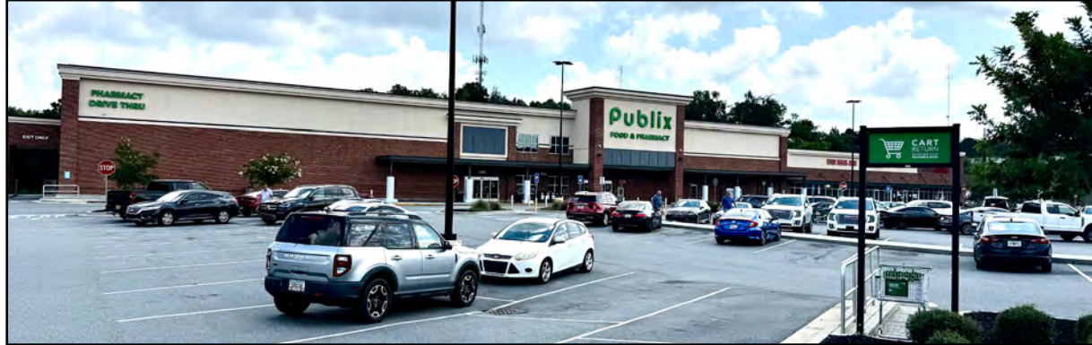
TOBESOFKEE CROSSING - PUBLIX - ADJACENT PROPERTY
